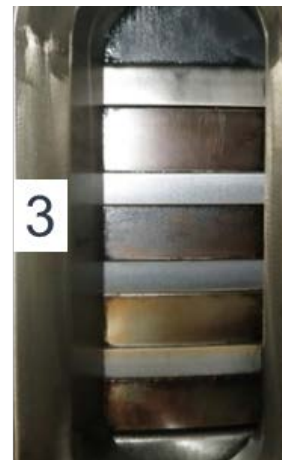
Same engine as opposite picture. Port inspection, cyl. 3. 2883 running h. Cylinder lube oil: 70 BN, high feed rate, ACC=0.40. Note: The cylinder lube feed rate is increased to sufficient level -> low wear and the lube oil has cleaned the ringlands.
