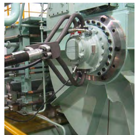
⑥ Hydraulic motor installed at the engine crankshaft
