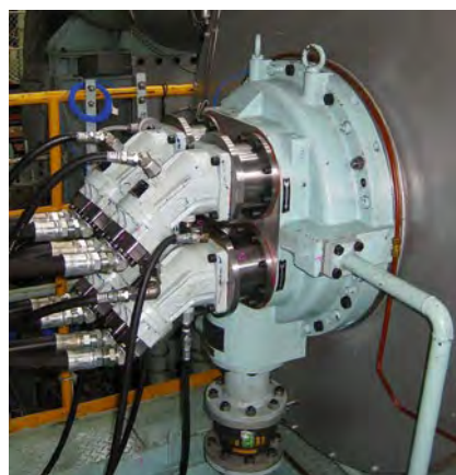
⑤ Hydraulic pumps installed at the turbocharger
